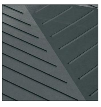
[1] GRAY TPO ROOFING MEMBRANE CONTOUR RIBS 16" O.C.
