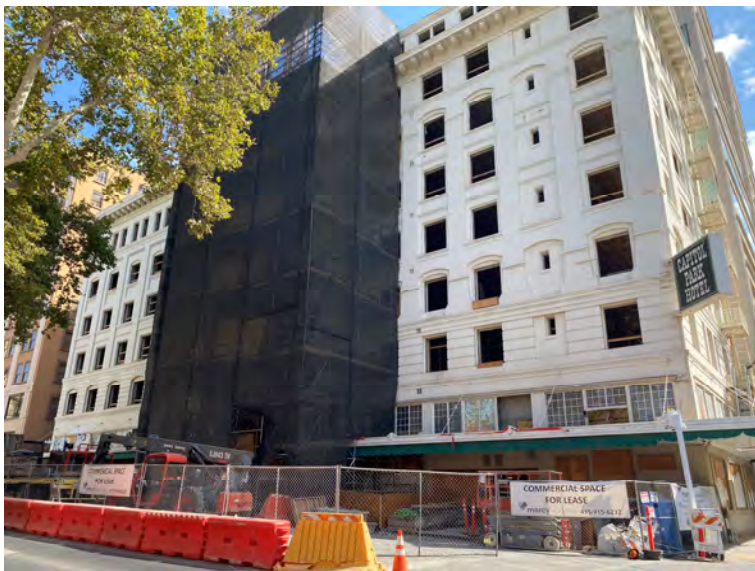
Capitol Park Hotel under construction
