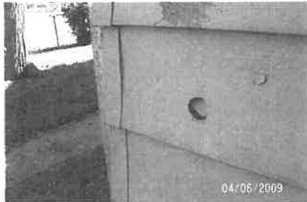
Picture #10 Holes drilled in exterior siding of house.
