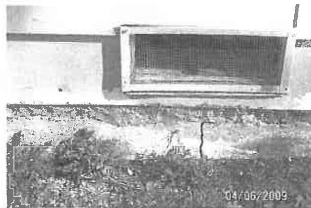
Picture #4 Exterior foundation crack
