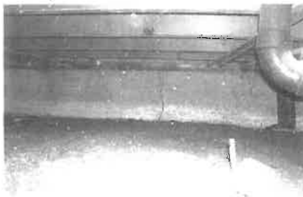
Picture #1 Crawl Space, Dry Rot, and foundation crack rear wall of home.
