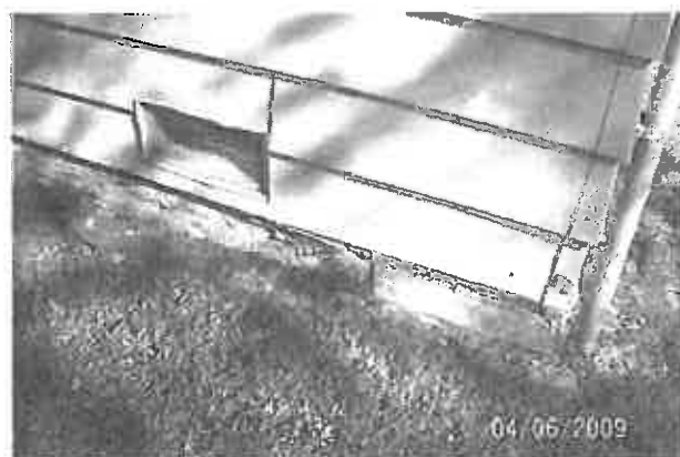
Picture #3 Exterior foundation crack and attempted repair
