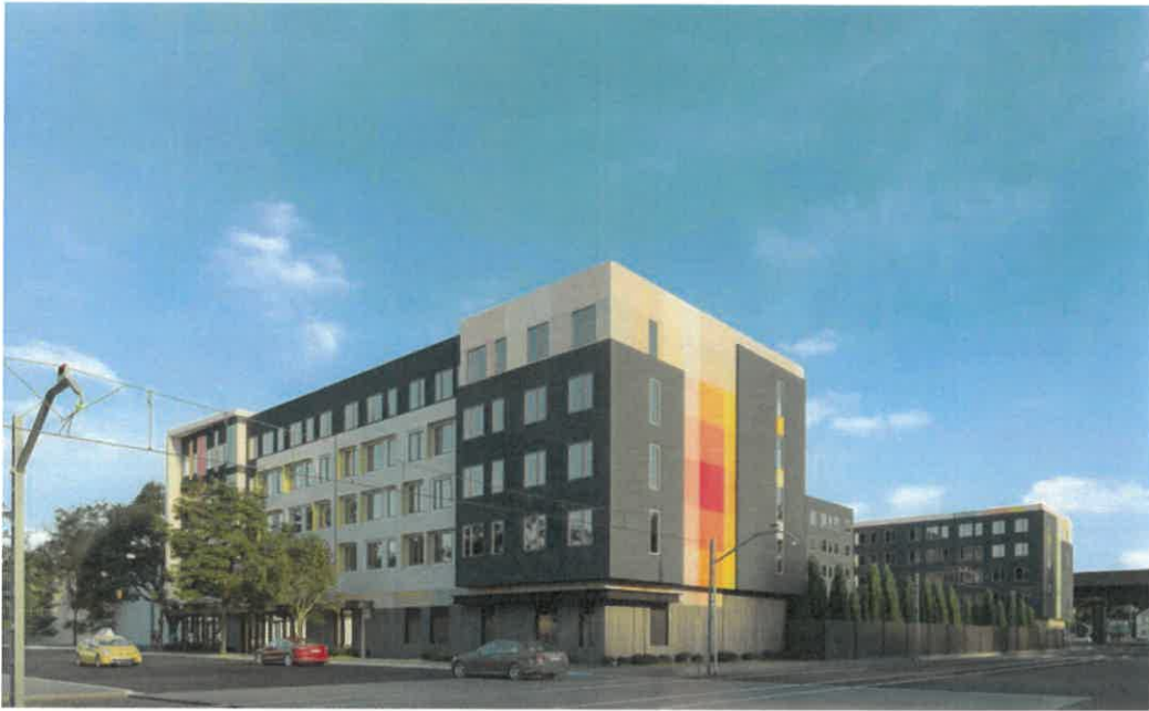
View from Broadway and Railway
