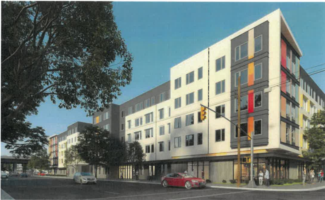
View from 19 th Street
