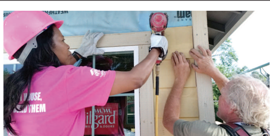
La Shelle Dozier helps build an affordable home during the Habitat for Humanity of Greater Sacramento annual Woman Build event.
