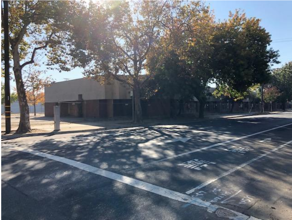
PHOTO #1. VIEW OF PROPERTY FROM 19 TH AND X ST INTERSECTION.
