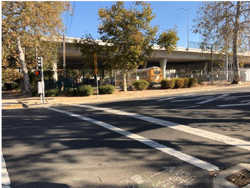
PHOTO #2. VIEW NORTH ACROSS X STREET TO BUS PARKING LOT.
