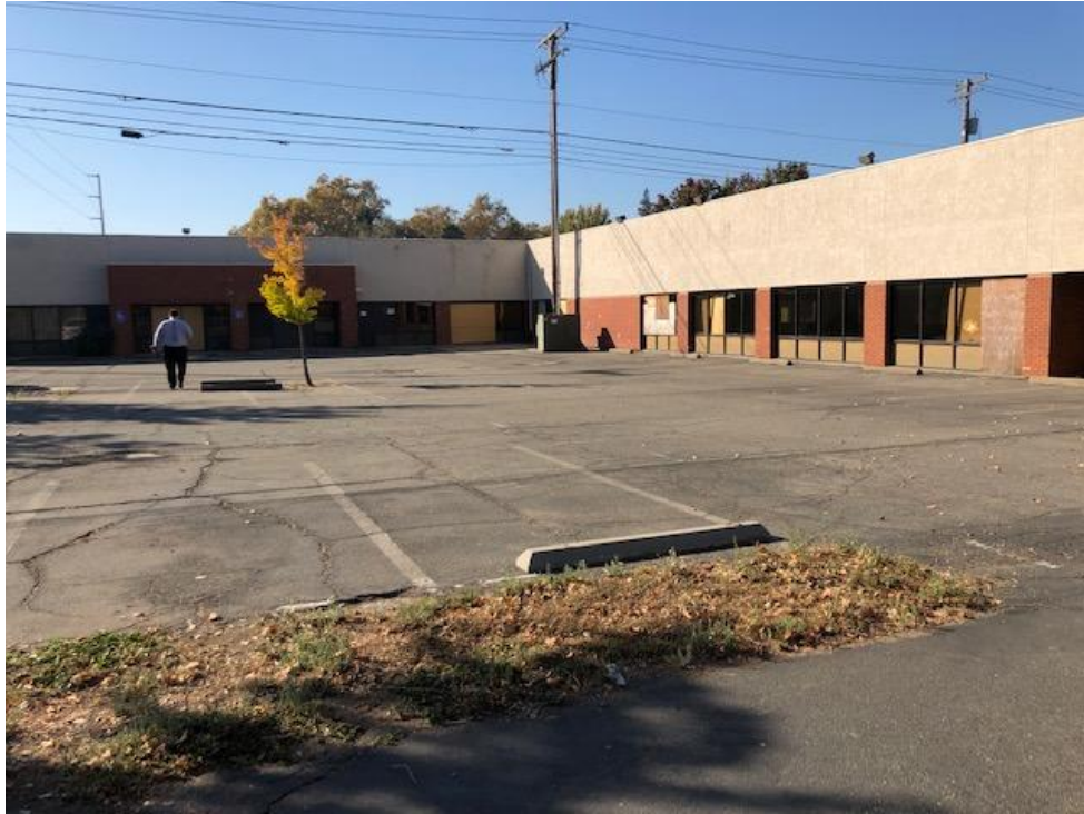
PHOTO #3. VIEW OF PROPERTY FROM ENTRY AND PARKING LOT.
