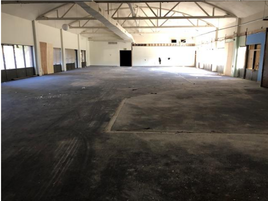
PHOTO #7. VIEW OF PROPERTY INTERIOR.
