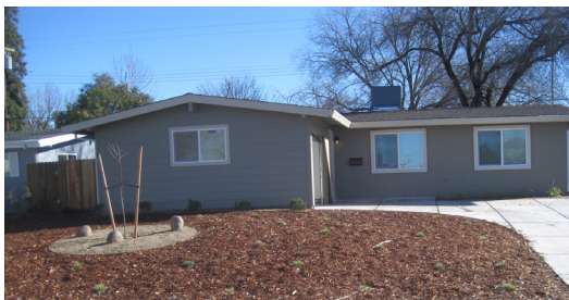
Left: A home before and after rehab.
