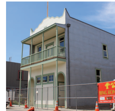
THE BING KONG TONG BUILDING RESTORATION The restoration of the Bing Kong Tong building in the city of Isleton is an important milestone in the ongoing efforts to highlight and preserve the historical, cultural and architectural contributions of the early Chinese settlers in the Sacramento River Delta. The building will be eventually used as a museum and community space.
