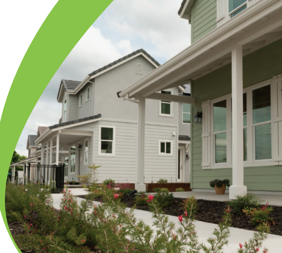
DEL PASO NUEVO DEVELOPMENT The completed Del Paso Nuevo development in North Sacramento will feature 300 high quality affordable single family homes. The benefits of the DPN project extend beyond the boundaries of the development into the surrounding community, including infrastructure, parks, commercial development and job opportunities.
