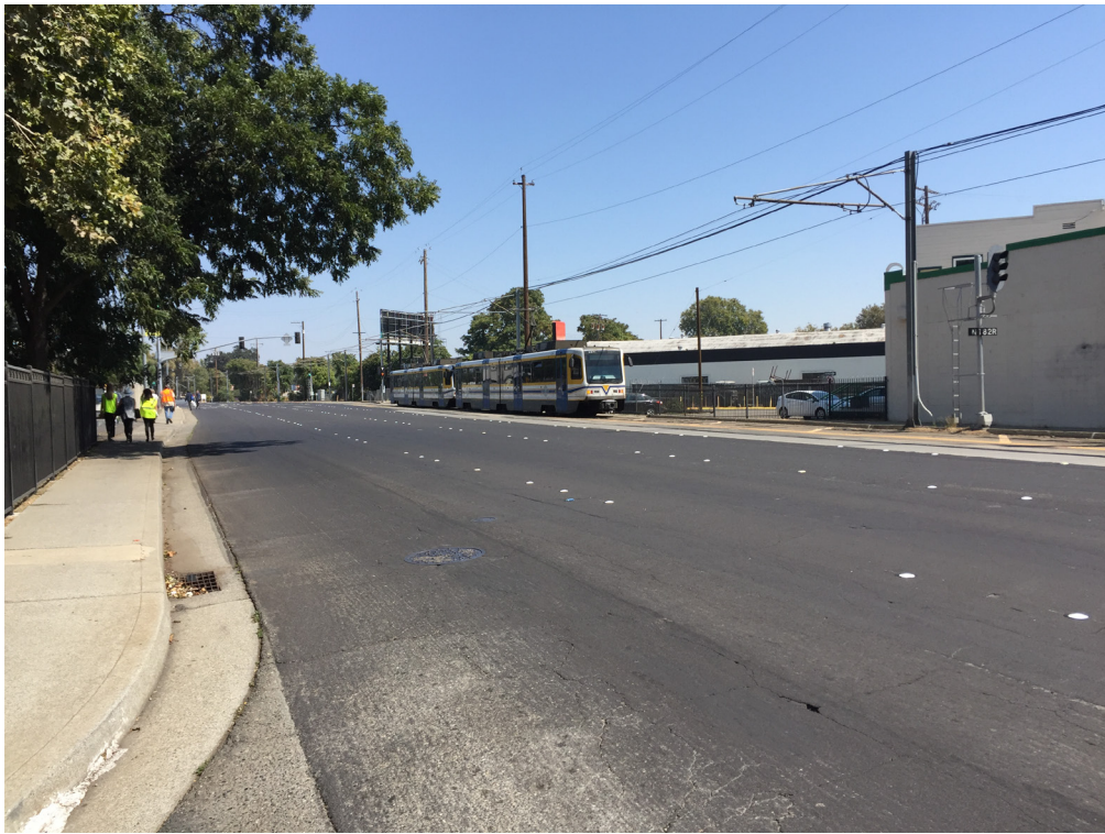
View looking north along North 12th Street, as viewed from existing Twin Rivers Community Housing Complex main entrance.
