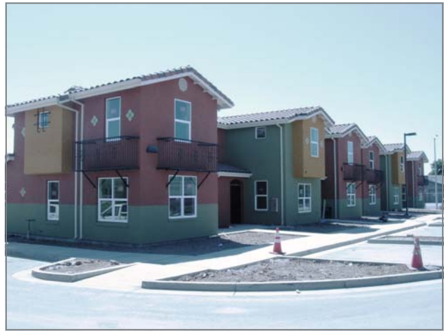
The new Colonia San Martin apartments near the Florin Mall Town Center are scheduled to be completed in November. The $76 million project will provide housing and onsite supportive services for low income individuals and families with HIV/AIDS.
