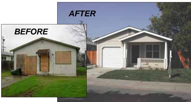
(Above) This house at 3721 17 th Avenue was enlarged from 749 square feet to 893 square feet. All three bedrooms in the one bathroom house were expanded and air conditioning was installed. Before rehab: Plywood siding with dry rot problems, aluminum windows, a small garage, non-descript elevation, cracked driveway, undesirable floor plan. After rehab: Varied siding materials, new bungalow-style elevation with covered porch, expanded garage, new driveway, re-designed floor plan, completely remodeled interiors, new landscaping.
