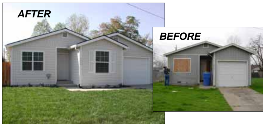
(Above) This three bedroom, one bathroom house at 4604 36 th Street was enlarged from 800 square feet to 985 square feet. A bonus room was added, the kitchen was expanded, and air conditioning was installed. Before rehab: Plywood siding with dry rot problems, aluminum windows, small garage, non-descript elevation, and cracked driveway. After rehab: Varied siding materials, new garage, existing garage converted to bonus room, completely remodeled interior, new driveway, new landscaping.
