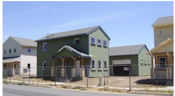
North Sacramento is the home of Surreal Estates, a new affordable live/work single-family housing community for artists. A grand opening is planned for September 2006.
