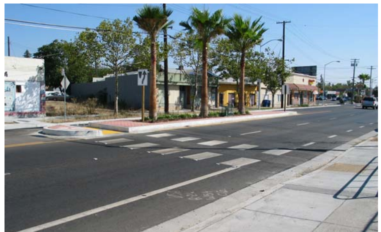
The award-winning Stockton Boulevard Beautification Project Improvements included landscaped medians, curb ramps, sidewalk, curb and gutter and related drainage improvements.
