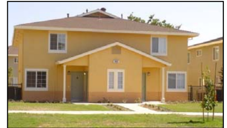
Phoenix Park apartments before and after reconstruction.
